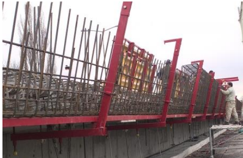
Bridge deck extension
