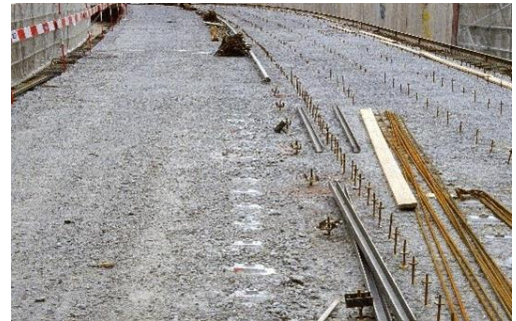
Bridge deck reinforcement
